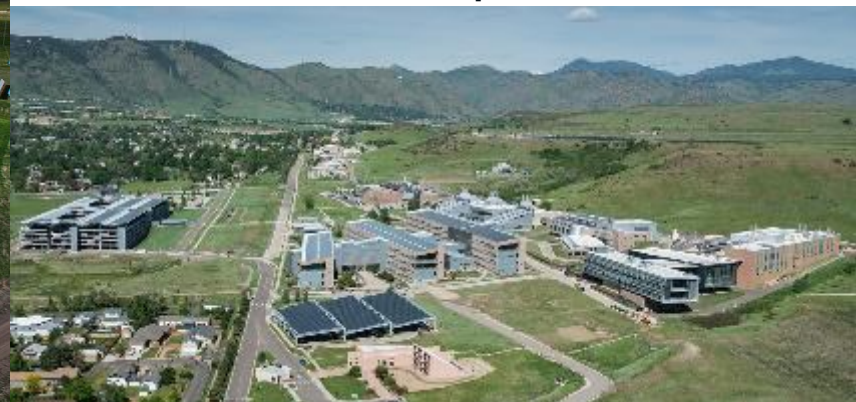
Main NREL Campus
